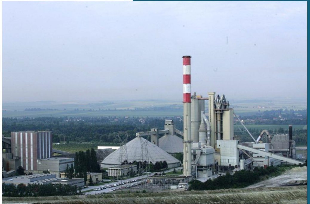
Usine de Couvrot (source : Ciments Calcia)
